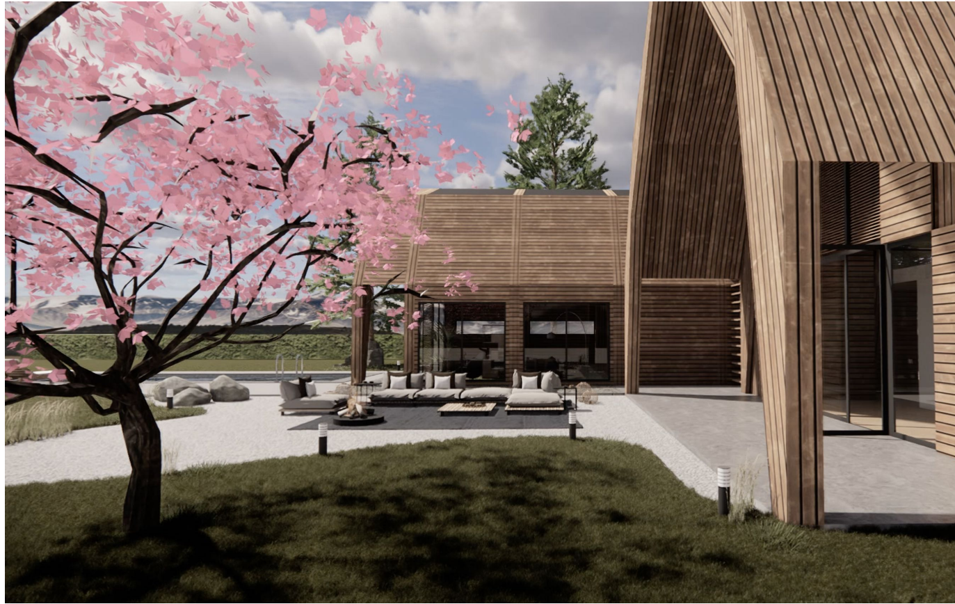
The verandas on the south-west facades offer shading and prevent overheating during summer
